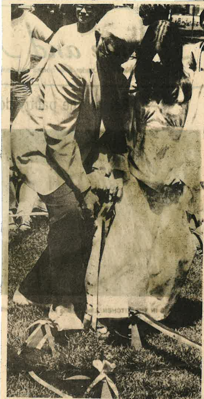
E.W. Harder, Garner-Hayfield elementary principal and Shelly Draper, bicentennial committee member, put the shovel to dirt readying the ground for the time capsule which will be buried and unearthed in the year 2026. Various items will be buried representing this era. When unearthed, future generations can read how life was back in the 20th century. [Leader Photo]
