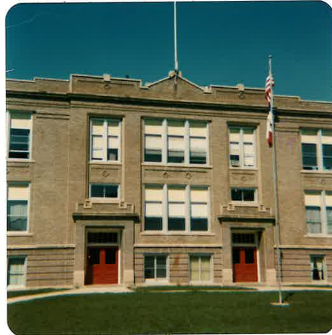
Garner-Hayfield Jr. High School Building 1976
